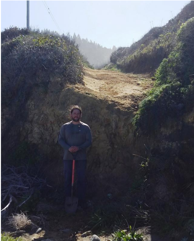
Figure 12. View southeast toward south bluff vertical access.
