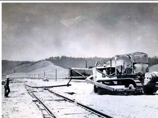
Removing rails in 1949, courtesy FB-MCHS.
