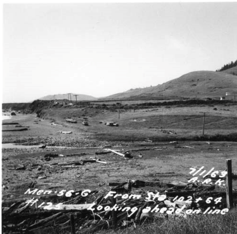
In this month's historic photo, here's the view north across the mouth of Dehaven Creek on July 1, 1963, before the new Highway One bridge was built. (Caltrans photo)
