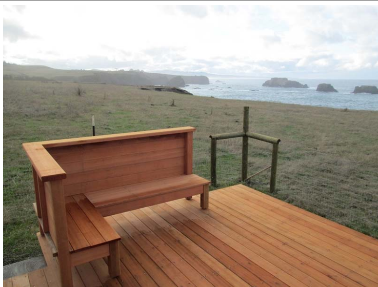
New Kibesillah Bluff Viewing Platform
