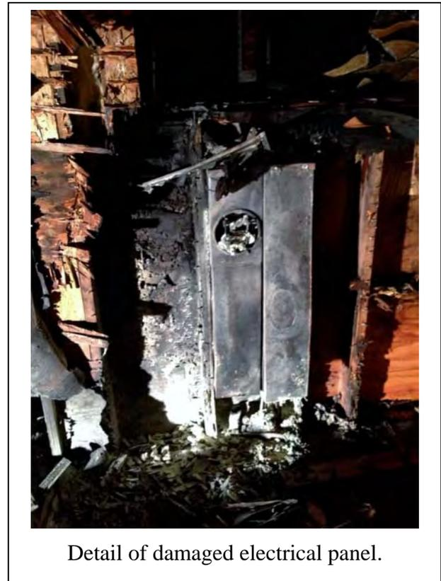
Detail of damaged electrical panel.
