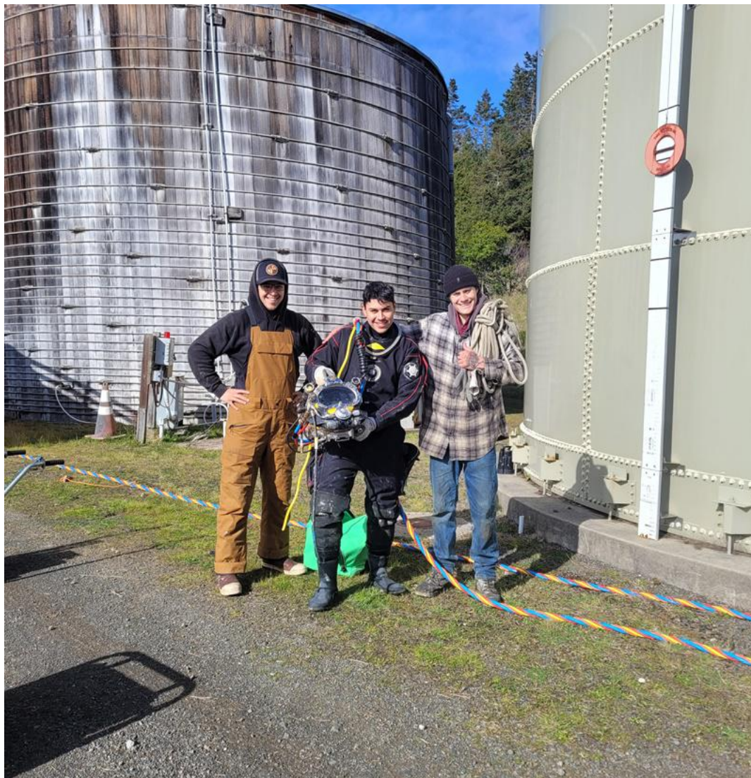
MIT Diving and Coating Crew servicing the Westport Water Storage Tanks: Left Steve Sanchez, Center Chris Rendon, Right Samuel Placek
