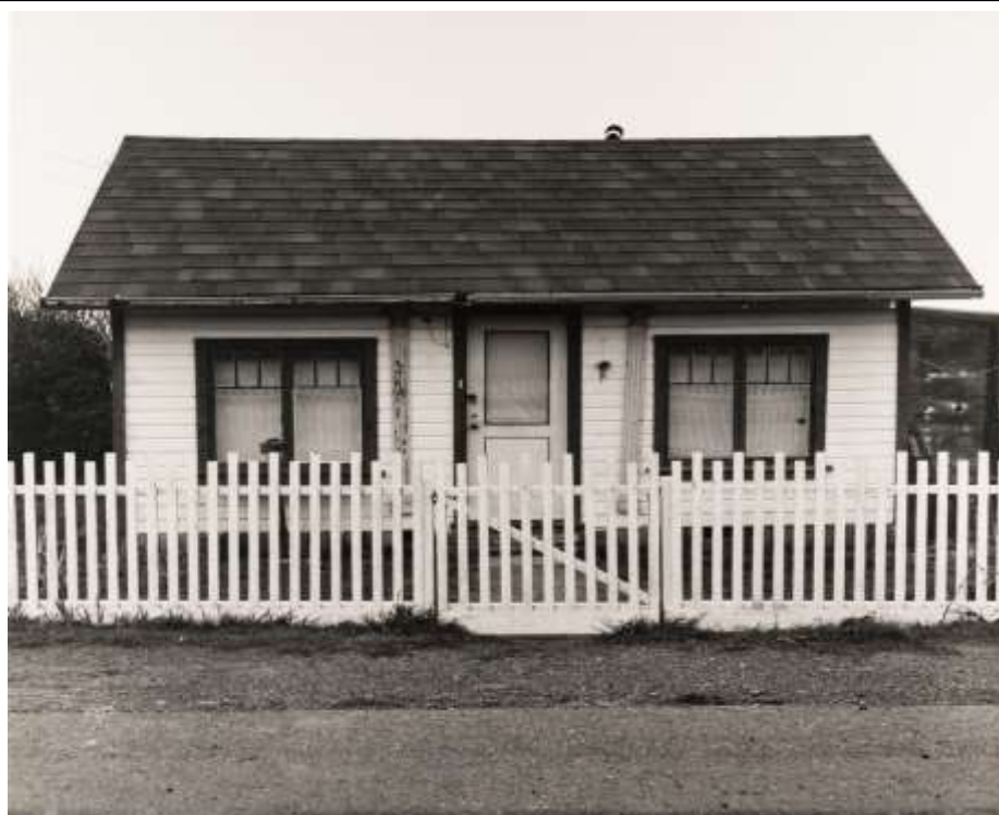
50 Years Ago, by Bill Brazill – This was Carl Harlison’s house in 1973 when Bill took this photo. It is the last house on the left along Highway 1 as you leave Westport Village going north, and is a perfect example of the symmetry and functionality of so many early homes.
