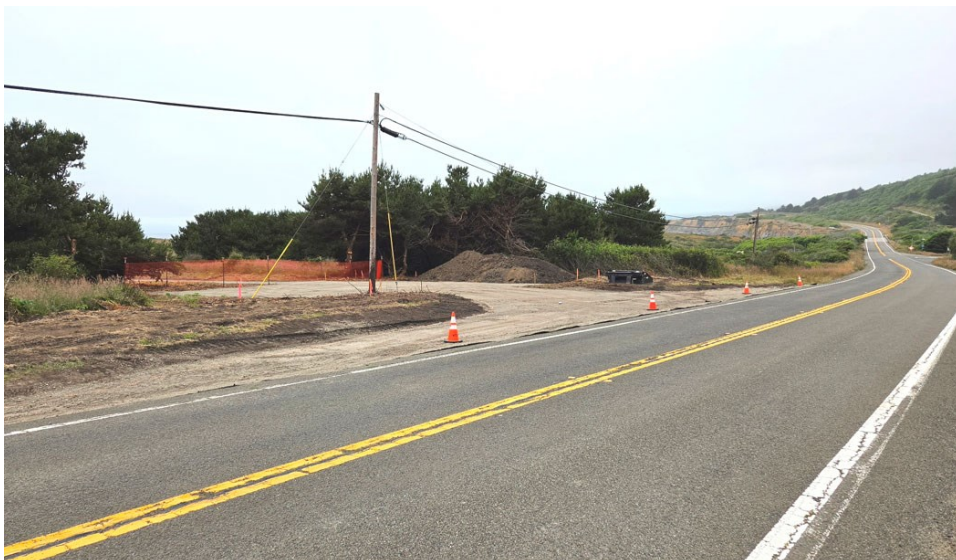
Work progresses on the DeHaven Headland parking area situated just south of DeHaven Beach and the Branscomb Road junction with Highway 1.
