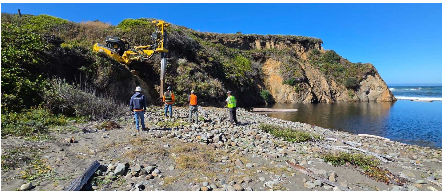
The drilling operation for the stairway being built on the south bluff next to DeHaven Beach. Work began on July 29. Work on the stairs will continue through August as WVS uses a grant from the State Coastal Conservancy to improve access to the 26 acre property.
