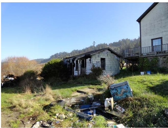
Old structure needing demolition and removal.
